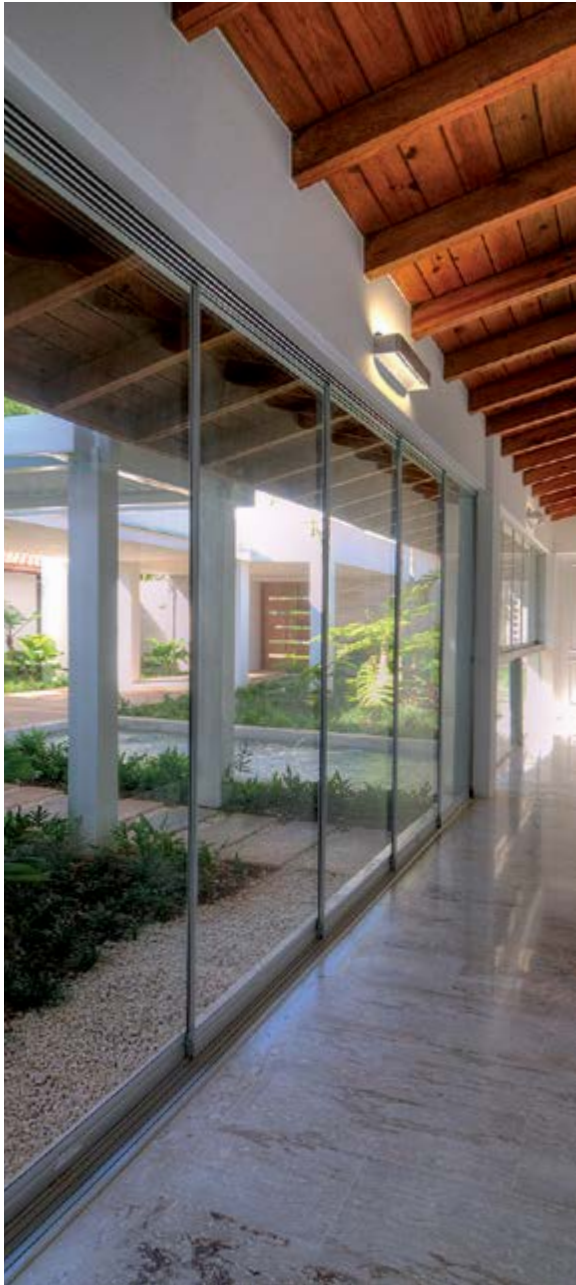
Cerramiento seeglass RUN 5 carriles / Glazing enclosure seeglass RUN 5 rails
